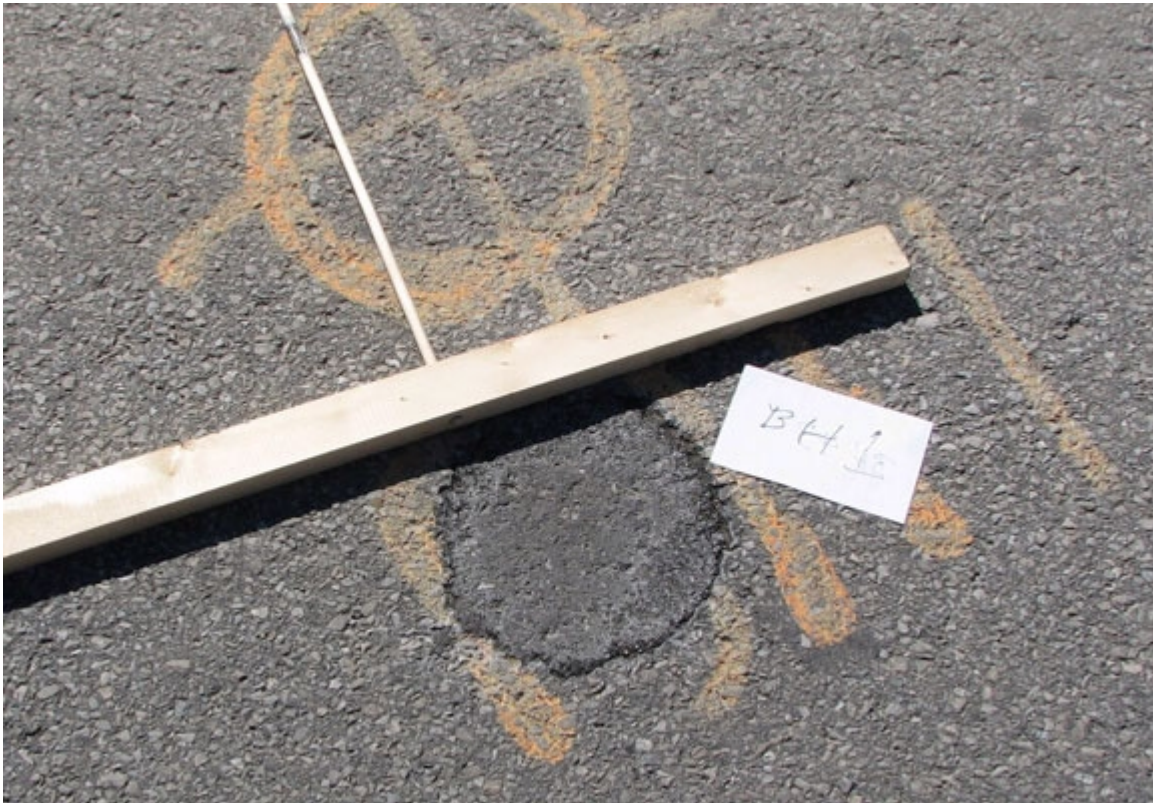
BH 43 is on the west side of Centre Road just at the bend north of the 11th. The depth is about 1/8"
